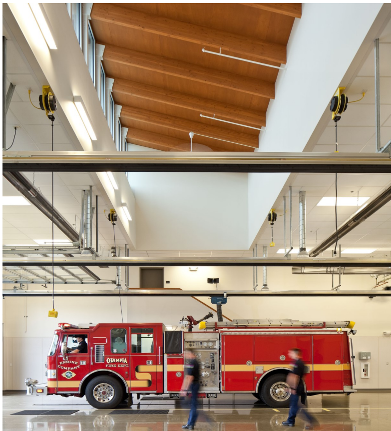
Beneficial clerestory daylighting in the apparatus bay of City of Olympia Fire Station 4.
